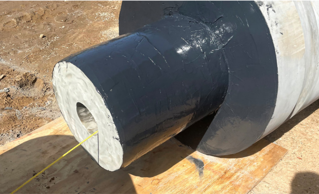
Belzona 2211 (MP Hi-Build) Flexible, multi-purpose rebuilding-grade polyurethane elastomer suitable for repair applications on rubber and metal components.
