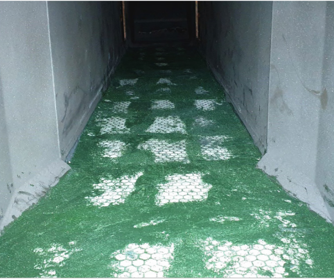
Belzona 1813 High-temperature, ceramic-filled abrasion and wear-resistant epoxy repair composite.
