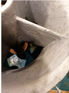
Belzona 1121 (Super XL-Metal) High-performance, extended working life, durable epoxy composite for the repair and rebuilding of metal components.
