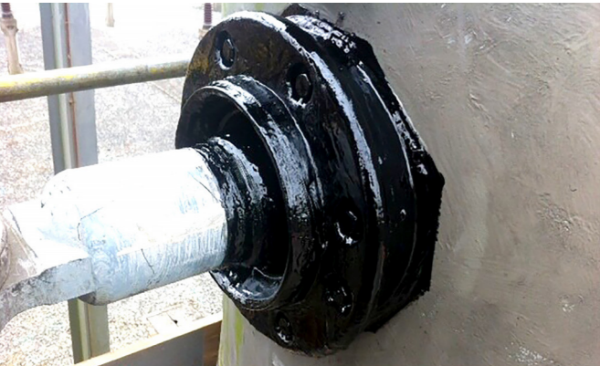
Belzona 2111 (D&A Hi-Build Elastomer) Flexible rebuilding-grade abrasion-resistant polyurethane elastomer, suitable for repairing damaged rubber and metal surfaces.
