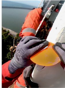
Belzona 5711 High-performance, solvent-free rebuilding material designed to spread damage to the leading edges of wind turbine blades.
