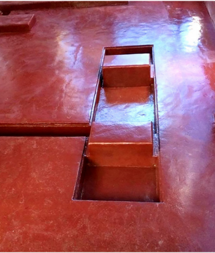
Belzona 4181 (AHR Magma-Quartz) Acid and heat-resistant epoxy concrete repair mortar.
