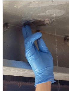
Belzona 9611 Rapid-curing system for the emergency sealing of low pressure leaks, prior to a more permanent repair.
