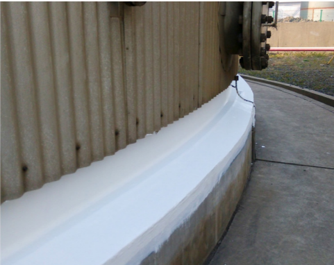
Belzona 3211 (Lagseal) Water-based, fire-resistant flexible membrane for the protection of all types of thermal insulation and cladding systems.
