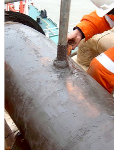
Belzona 1251 (HA-Metal) High-performance, heat-activated epoxy repair composite for applications directly onto hot metal surfaces.
