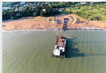
Barge GAVERLAND dredged a 750m trench and assisted in installing high-voltage cables at the Saint-Nazaire wind farm.
