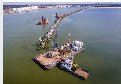
ALBATROS and GAVERLAND placing rocks for the renovation of a breakwater in Klaipeda, Lithuania.
